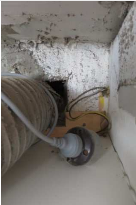
"A" unit flexi duct into "B" laundry
