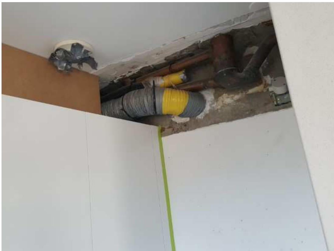
"A" unit flexi duct into "B" laundry
