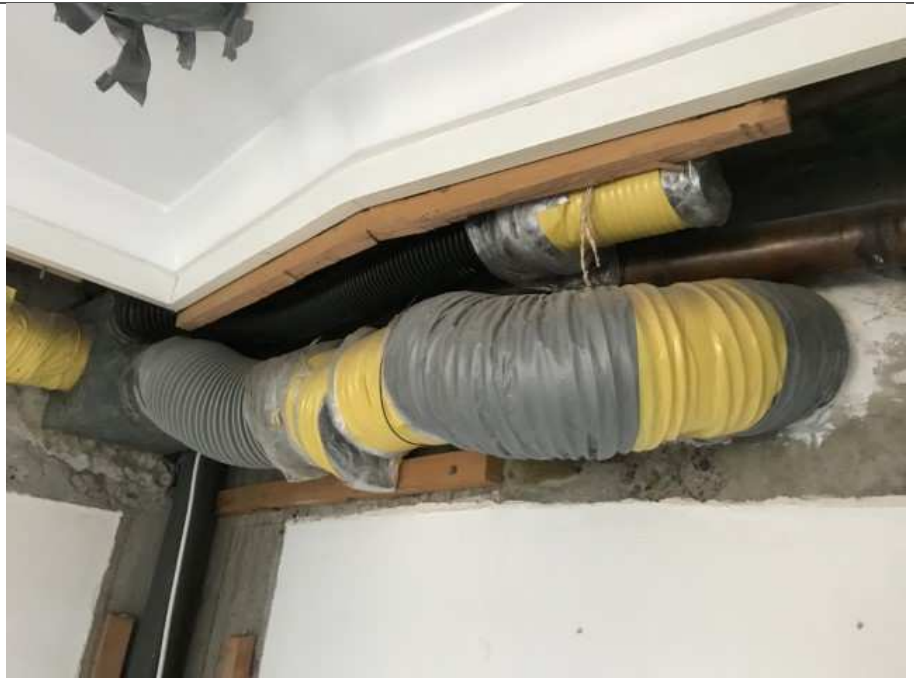
"B" laundry. Plenum chamber on left, "A" exhaust duct. See Note 1 below.
